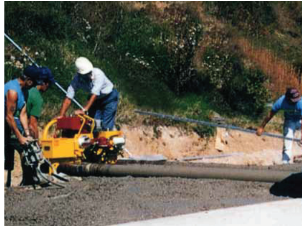
The Roller Screed does a great job on many types of concrete finishing such as roads, runways, bridges, inclines, etc.
